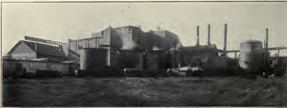
A PARTIAL VIEW OF THE WORKS OF THE PATERSON MANUFACTURING COMPANY, LIMITED.
